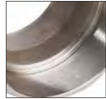
Socket weld connection
